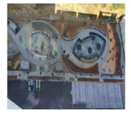
Climbing wall RCC work completed & plastering work in progress, Amphitheater plastering completed, granite WIP, Clubhouse drain cutting work WIP, open Amphitheater Opposite club house block work WIP.
